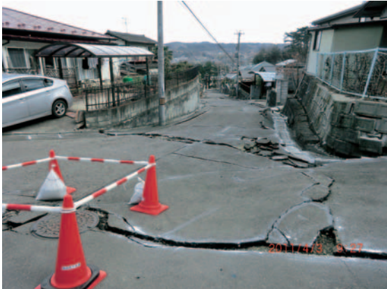
Fig. 3-14 A view of typical damaged houses in hillside residential areas, Oritate, Aoba District, Sendai City (Kazama, M.)
