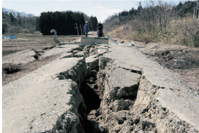
Fig. 3-31 Damage to a main agricultural pipeline for a length of about 1.4 km due to uplift caused by liquefaction of backfill soil. The largest depth of opening was about 1.6 m (Mohri, H.)
