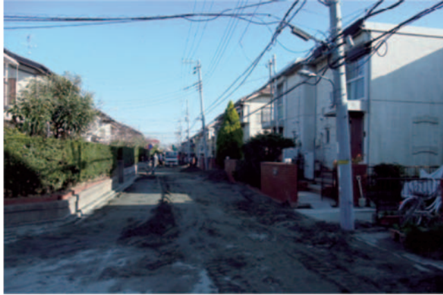
Fig. 3-18 Damaged houses and road due to soil liquefaction (Yasuda, S.)
