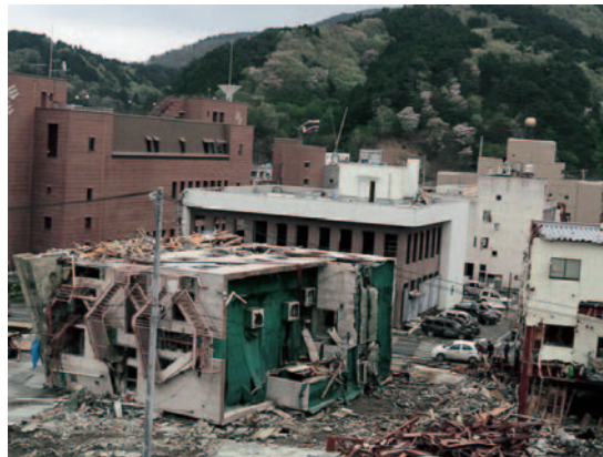
Fig. 3-10 A RC building over-turned by tsunami, Onagawa (Kodaka, T.)
