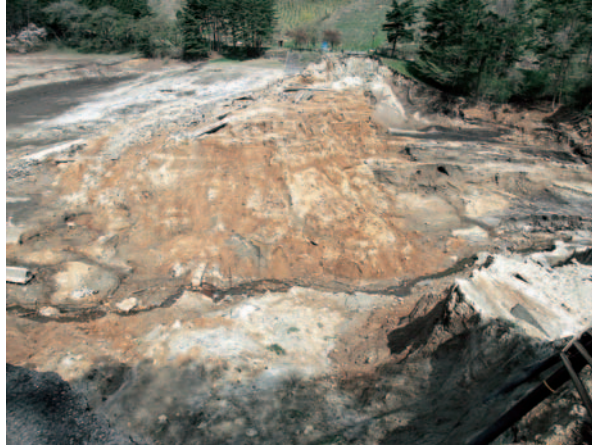
Fig. 3-4 Failure of Fujinuma dam in Sukagawa City, Fukushima Prefecture (Yasuda, S.)
