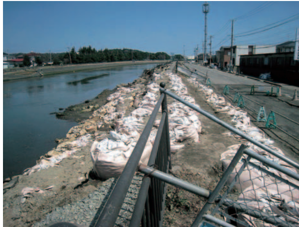
Fig. 3-30 Damage to river dike on the right bank of Sunaoshi River caused by earthquake motion, Tagajyo City, Miyagi Prefecture, and resulting inundation of lowland by tsunami (by Uzuoka, R.)
