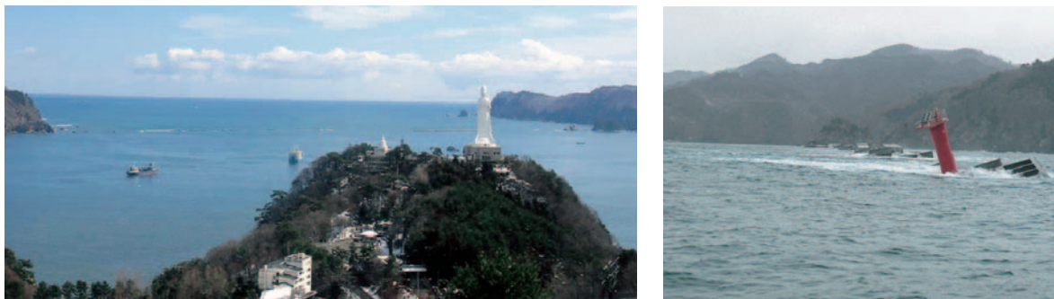
Fig. 3-6 Damage to a breakwater by tsunami at Kamaishi Port (by the courtesy of PARI)
