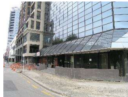
Figure 11 Earthquake damage to a well-designed building (sinking and tilting) caused by unsatisfactory subsoil condition
