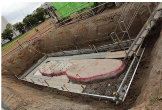
Figure 6 Geotechnical support for people's recovery from earthquake disaster (technical development of underground grid walls in liquefaction-prone soil)
