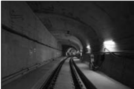
Kwun Tong Line Extension Contract No.1001, Yau Ma Tei to Whampoa Tunnels and Ho Man Tin Station
