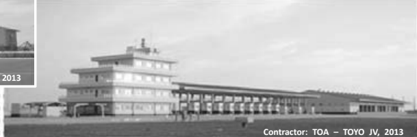
Contractor: TOA – TOYO JV, 2013
