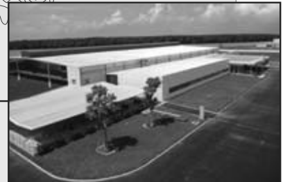
Paramount Bed Vietnam Factory Project
