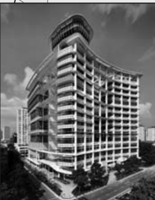
Singapore National Library Construction
