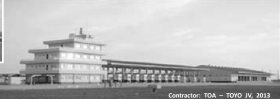
Contractor: TOA – TOYO JV, 2013
