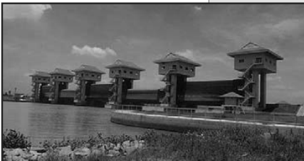
The Bang Pakong Diversion Dam
