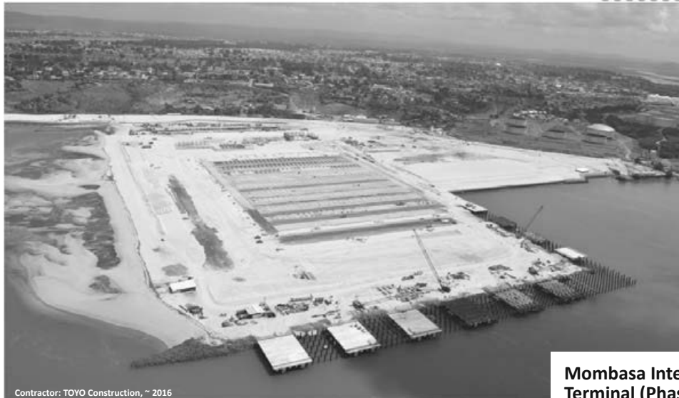
Contractor: TOYO Construction, ~ 2016
