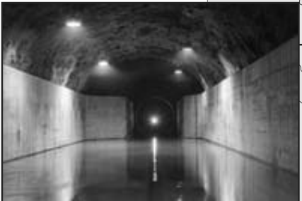
Pahang-Selangor Raw Water Transfer Project Lot 1-1 Water Transfer Tunnel and Related Works
