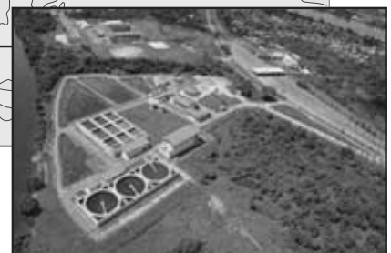
Centralized Sewerage System for Kuching City Centre (Package 1)
