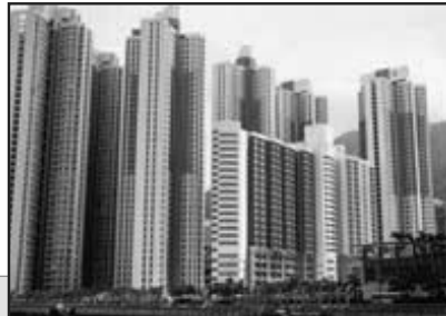
Aldrich Bay Development Work, Phase 4
