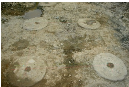
Fig. 1 Cement-treated piles
