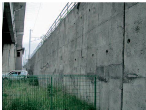
Fig. 2-8 Geosynthetic-reinforced soil retaining wall have a staged constructed full-height rigid facing for Tohoku line (railway), next to Natori River bridge, Sendai City; any damage by this earthquake (photo. by Okamoto, M.)
