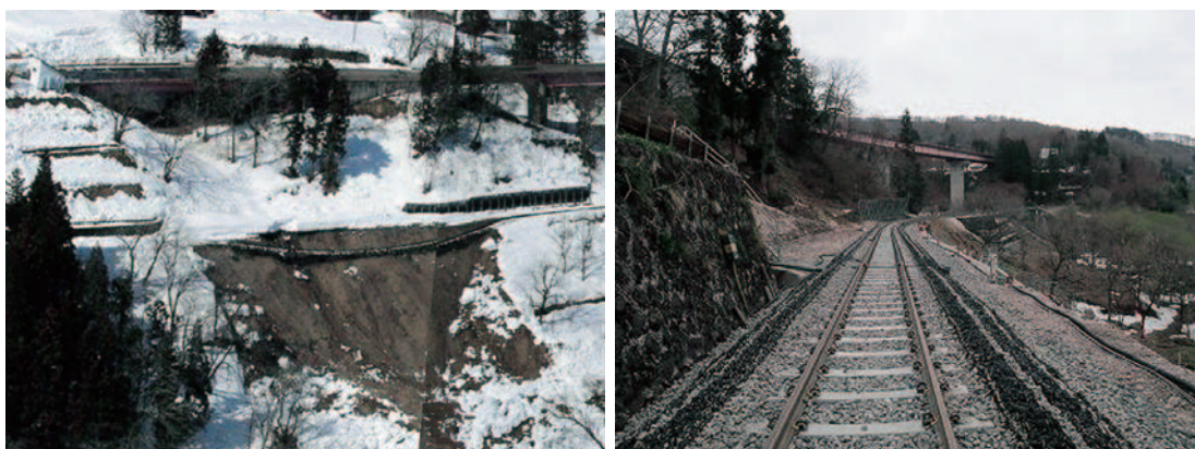
Fig. 3-12 a) Embankment collapsed in the Nagano-Niigata Border Earthquake induced the next day after the 2011 Great earthquake; and b) reconstruction to embankment retained by a GRS-RW having a FHR facing, between Yokokura and Morinomiya, JR East Iiyama Line (by the courtesy of the East Japan Railway Co.)
