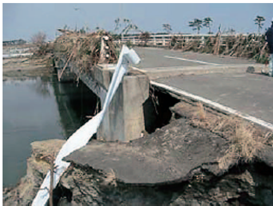
Fig. 11 Erosion of embankment at bridge abutment after tsunami Strike (Iwanuma in Miyagi Prefecture)
