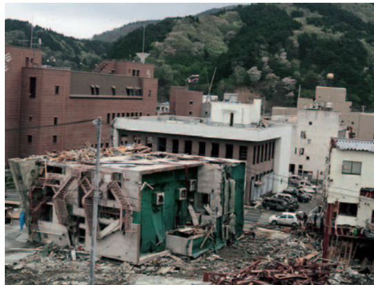
Fig. 3-10 A RC building over-turned by tsunami, Onagawa (Kodaka, T.)
