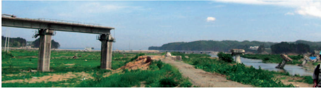
Fig. 3-9 a) Collapse of river dike in the upper reach of a bridge abutment on the left bank of Tsuya Rive, Motoyoshi, Kesen-numa City, Miyagi Prefecture (Uzuoka, R.) : b) a view from the upstream of Tsuyagawa Bridge, between Motoyoshi and Rikuzenkoizumi stations, Kesen-numa line, East Japan Railway: several girders were washed away and piers in the river tilted by tsunami (Tatsuoka, F.)
